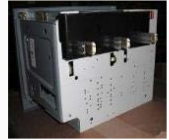
Rear view of bucket with stab assembly
