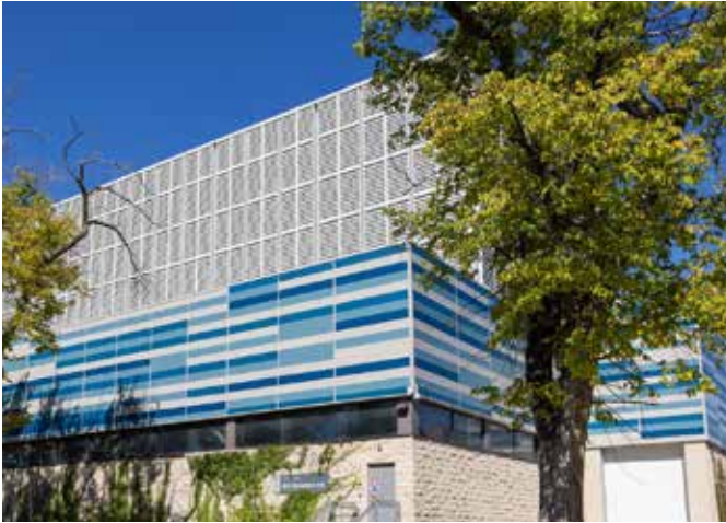
▲ The new 35,000-square-foot energy plant at Health Sciences Centre in Winnipeg was built with 4,500 tonnes of cooling capacity and 6 megawatts of emergency electrical power generation.
