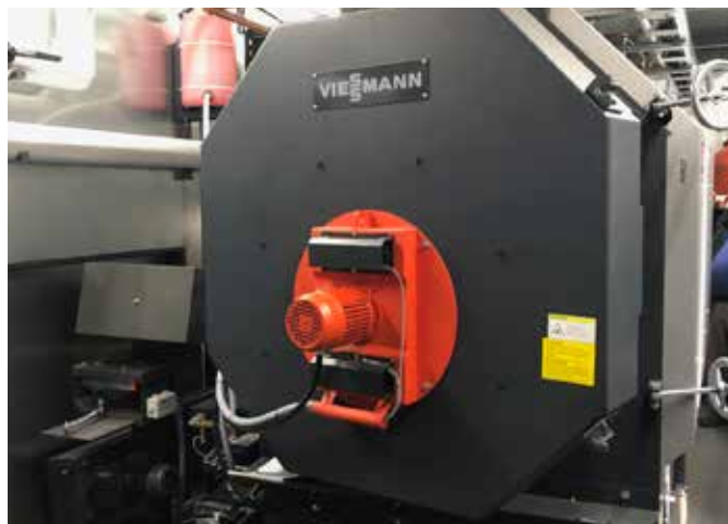
▲ The addition of the biomass plant, which works in tandem with the propane plant and carries up to 95 per cent of the space heating load, is projected to offset 6,200 gigajoules of propane each year.
