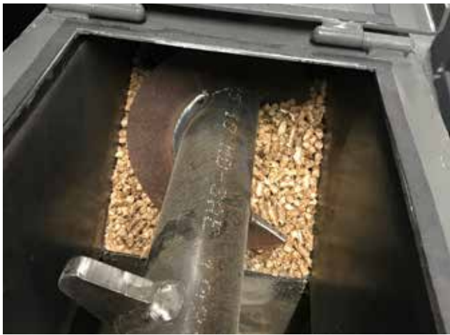
▲ The new plant's fuel source was originally supposed to be only wood pellets; however, to future-proof the plant and increase the resiliency of the fuel supply chain, a change had to be made to allow the silo and auger to accept both wood chips and pellets.
