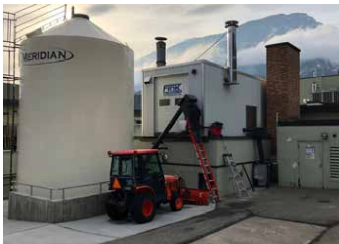
▲ The addition of the biomass plant, which works in tandem with the propane plant and carries up to 95 per cent of the space heating load, is projected to offset 6,200 gigajoules of propane each year.
